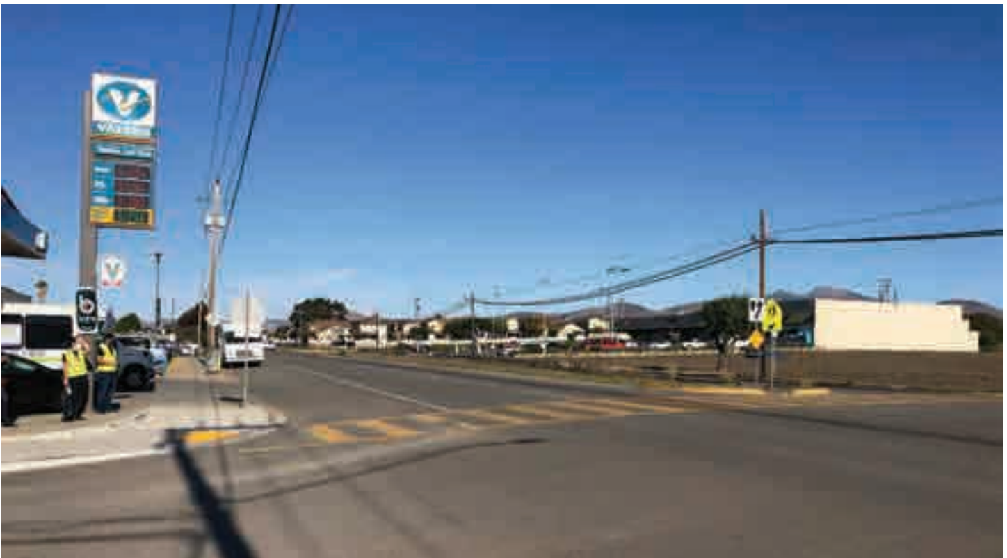
The crossings of San Juan Grade Rd were identified as a safety concern
