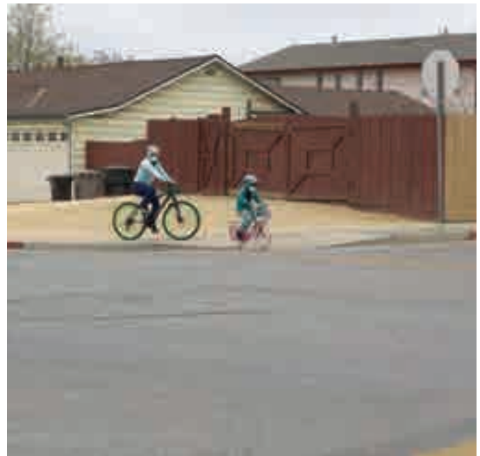
Bike lanes are recommended on Towt St between Freedom Parkway and Paseo Grande
