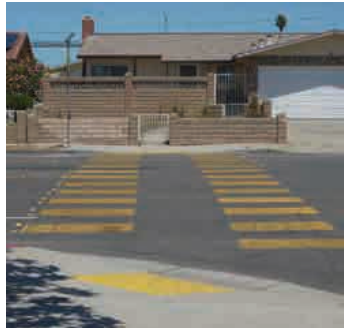
A high-visibility crosswalk was installed across E Alvin Dr at Modoc Ave
