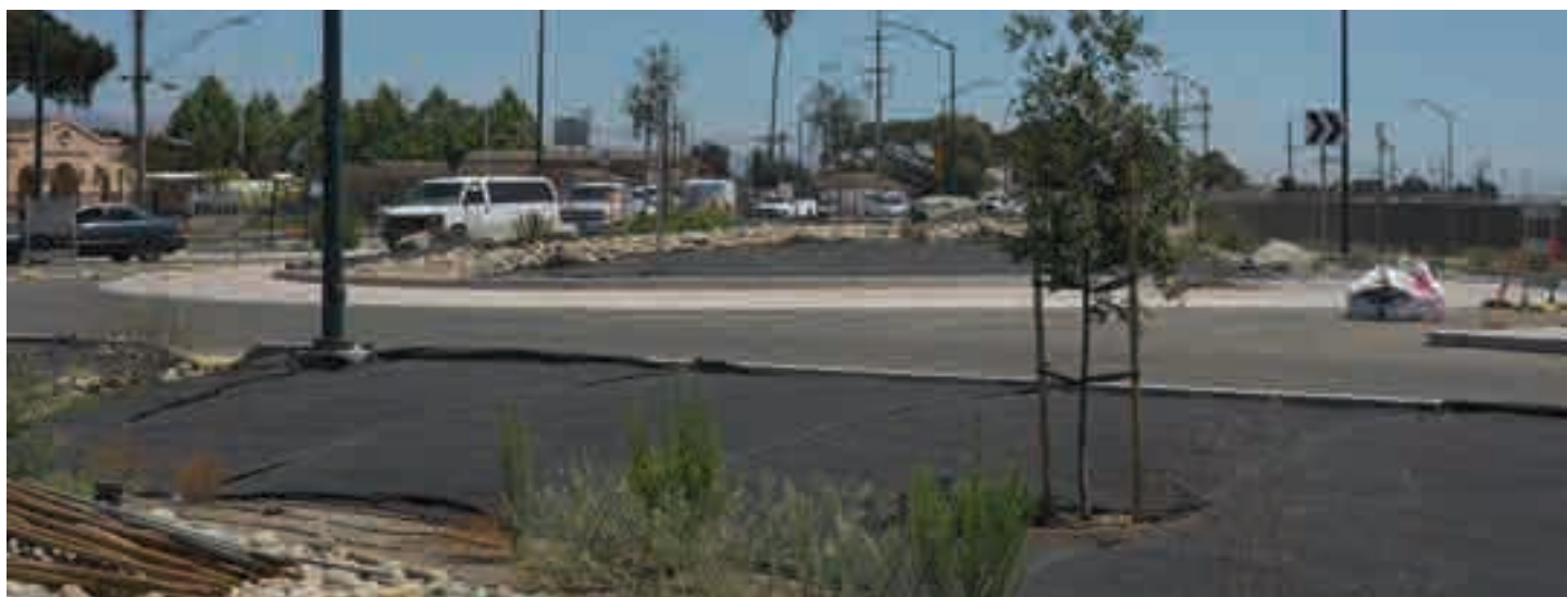
Roundabouts are currently in construction near Bardin Elementary.
