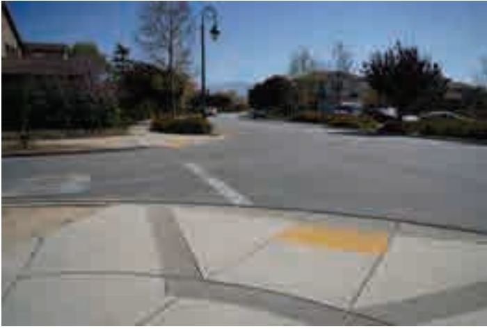
ADA compliant curb ramps near Monte Bella Elementary
