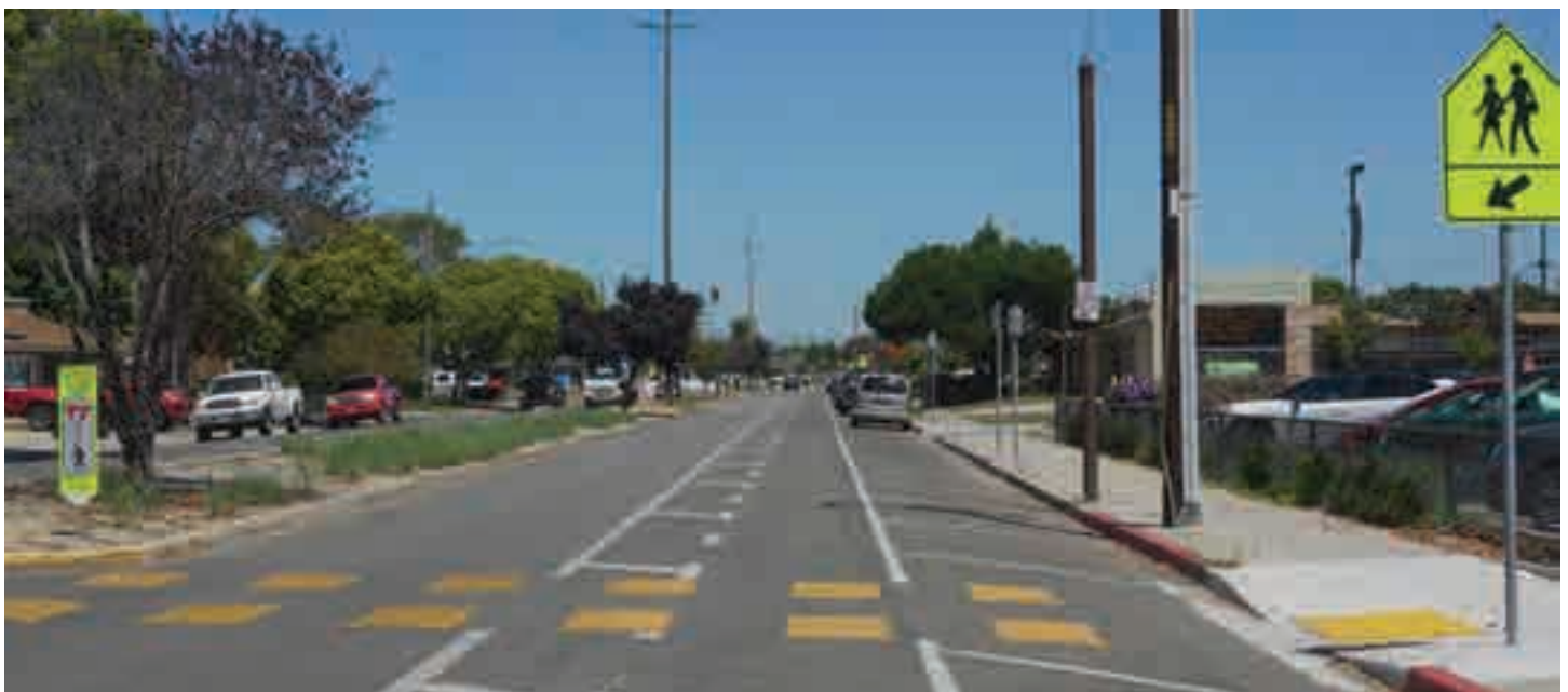
Buffered bike lanes and high-visibility crosswalks were recently installed on Linwood Drive
