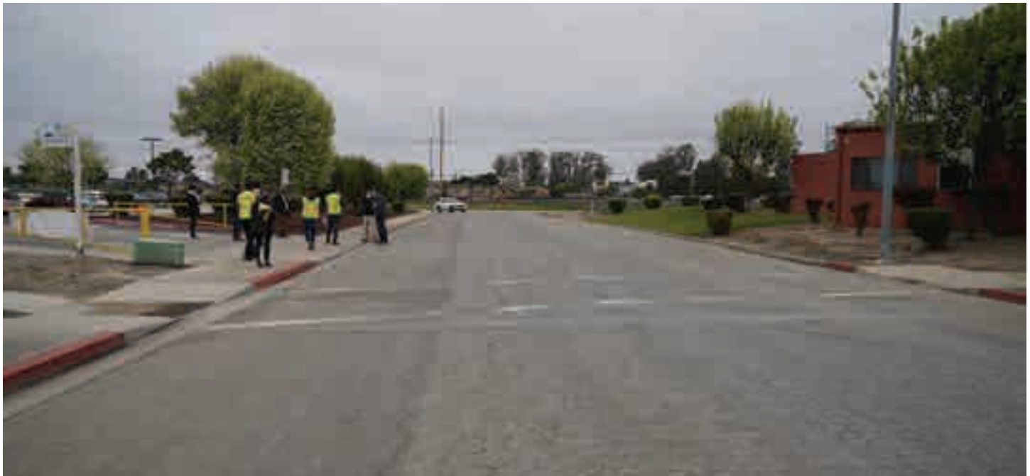
There is missing sidewalk on the north side of Sherwood Place
