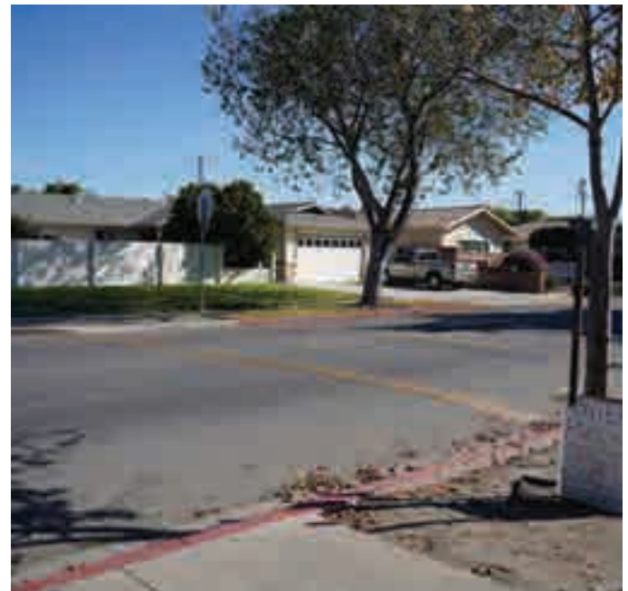
Curb extensions and high-visibility striping are recommended for the crosswalk in front of the school
