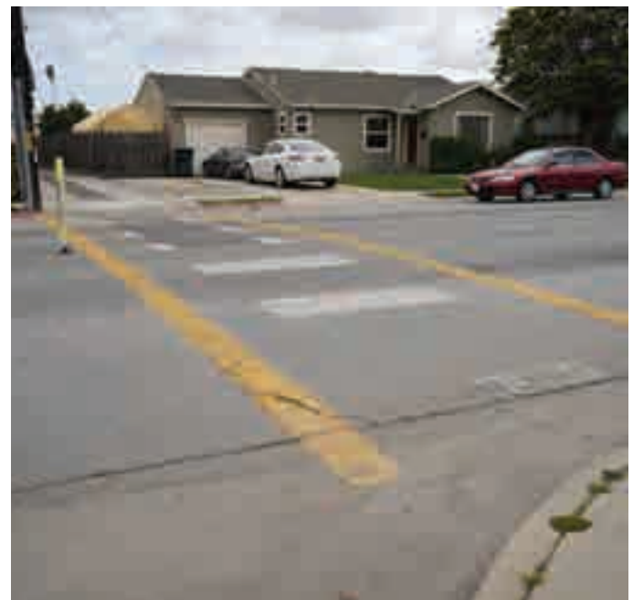
Curb extensions are recommended for the crosswalk at Towt St and Kentucky Ave
