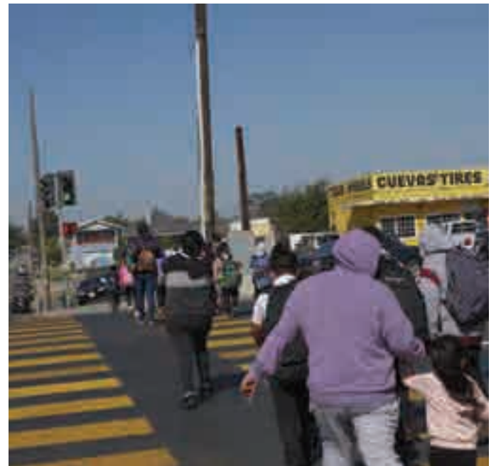
High-visibility crosswalks were installed on E Alisal St as part of the temporary installation project
