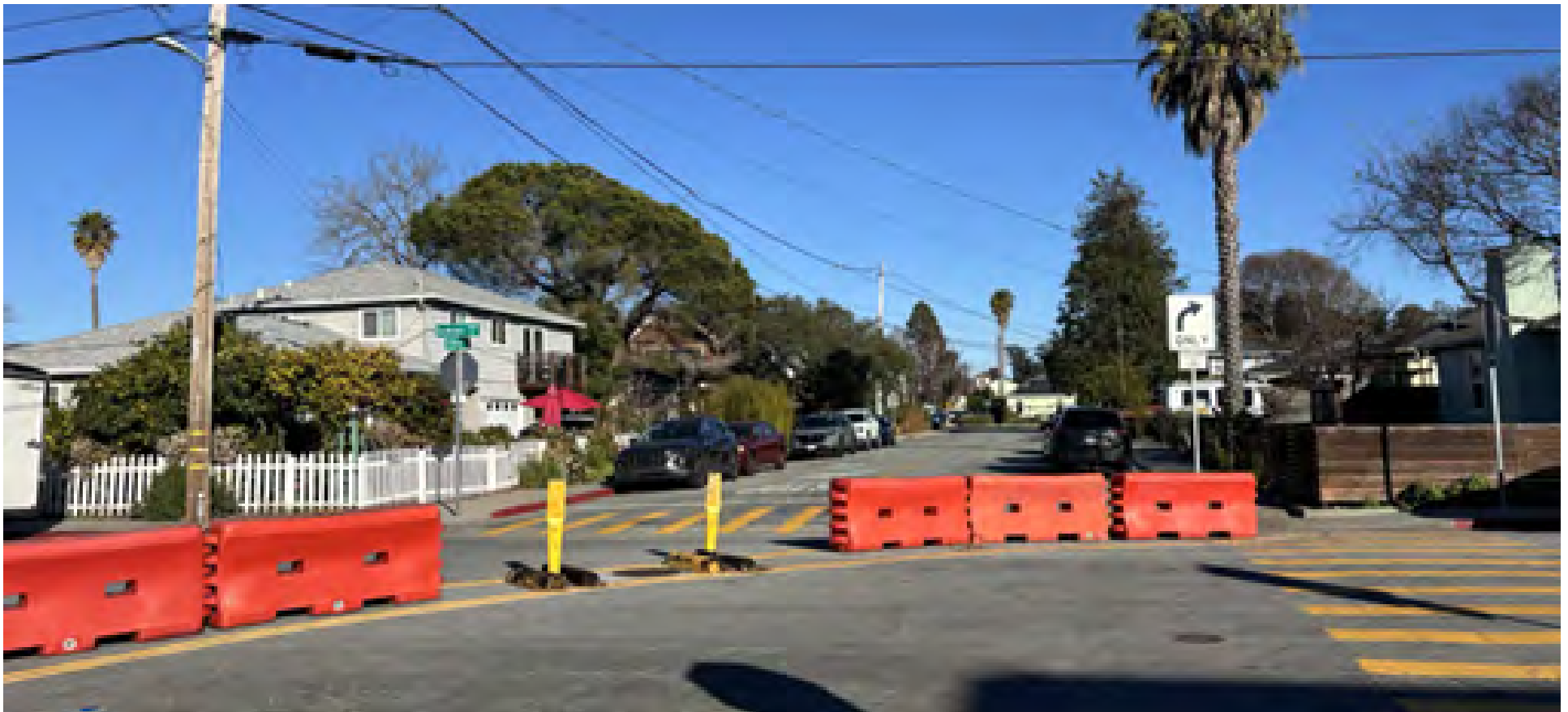
Figure 29. The City installed a quick-build traffic diverter at Summer Street and Effey Street.
